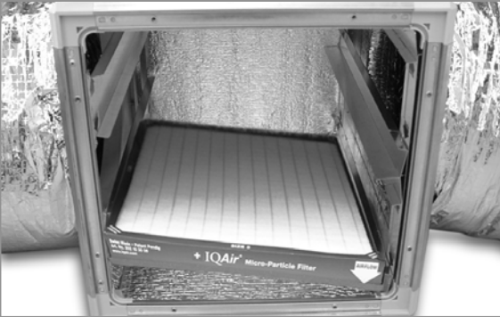
5. Insert new filters starting from the bottom.
