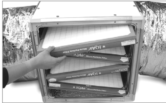
4. Remove filters starting from the top.
